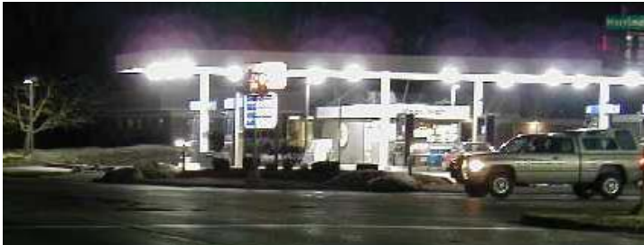
Photo A. Poor lighting
