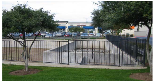
Facility that complies with current requirements, but not with proposed SM-1.
